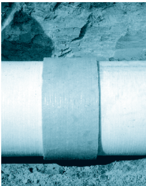
Figure 8-5 Joint à bride incorporé
